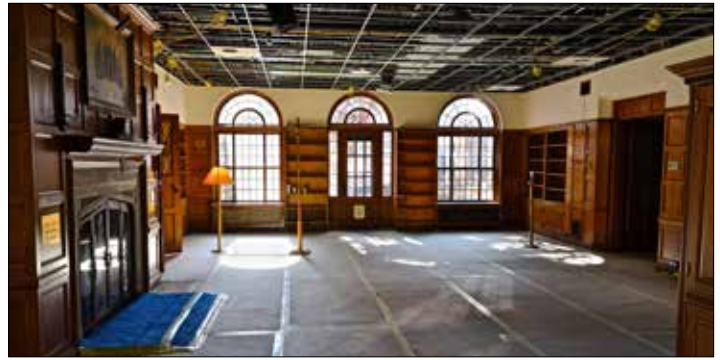
The library in process of restoration.
