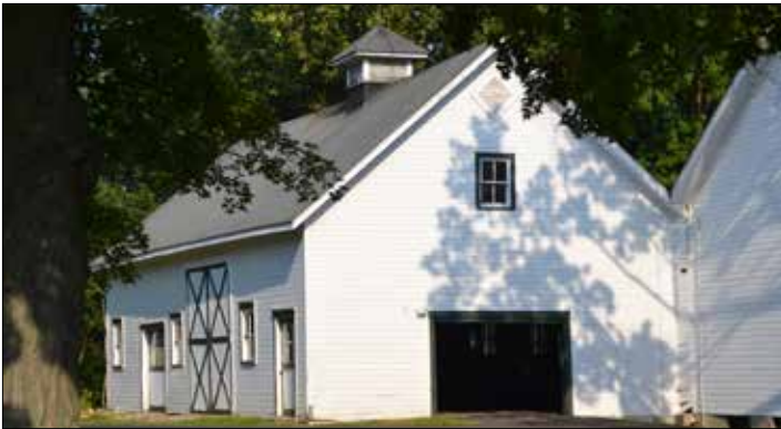
This photo was taken before last year's barn fire. Now an empty space awaits the construction of a new barn planned for later this year.
